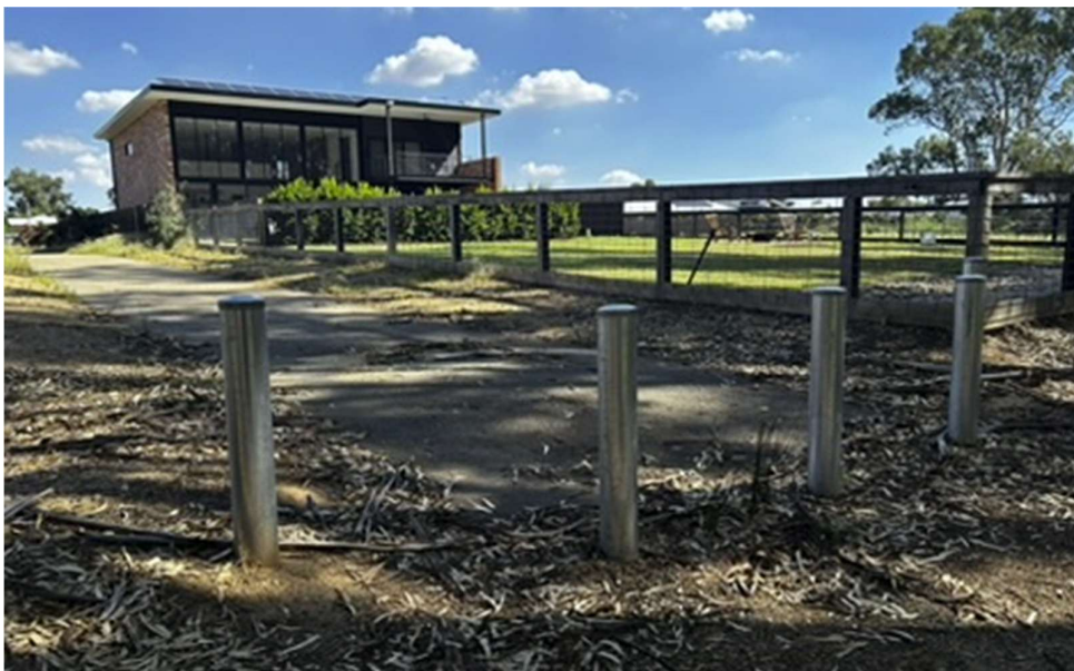
Pedestrian Access to the Foreshore area in Bundalong
