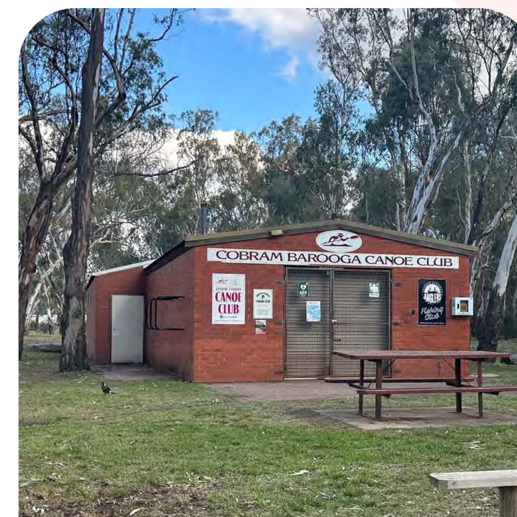
Existing Canoe Club - upgrades/storage required
