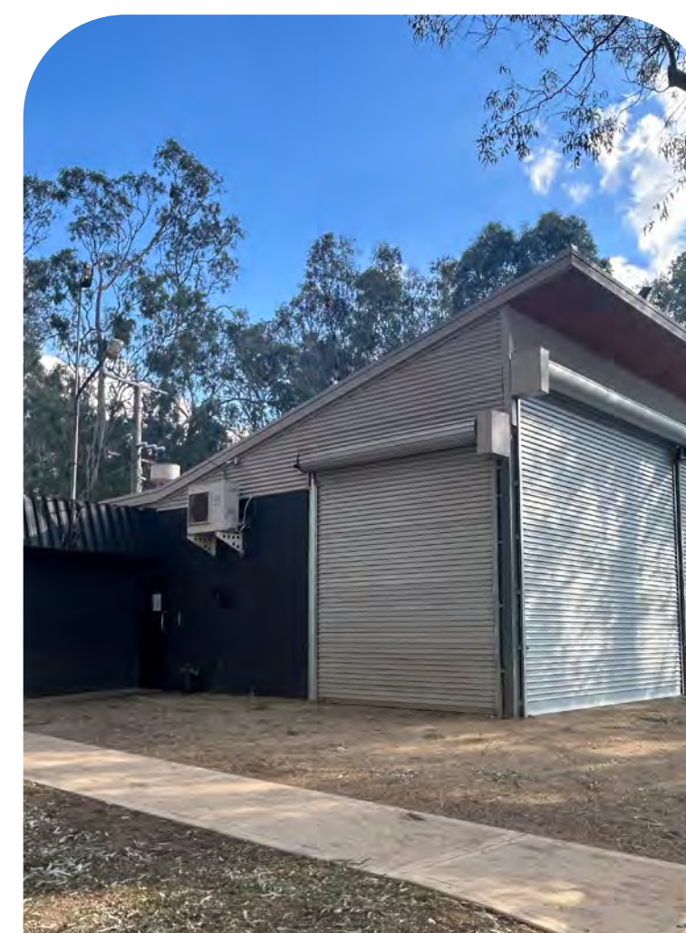
Existing cafe river frontage / dining
