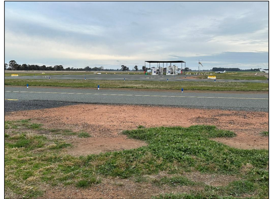
Figure 17 Aircraft refuelling facility
