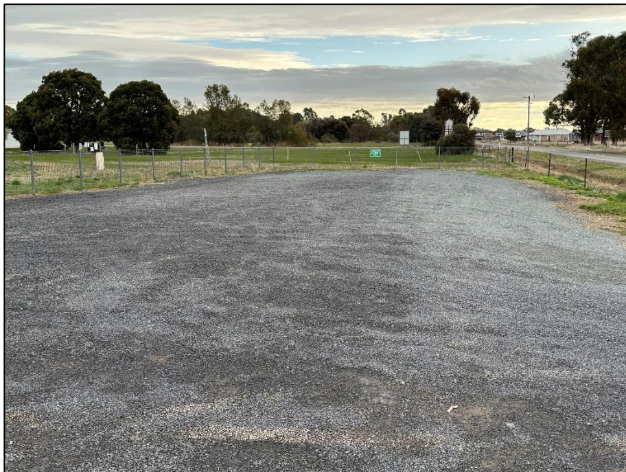
Figure 22 Terminal car park
