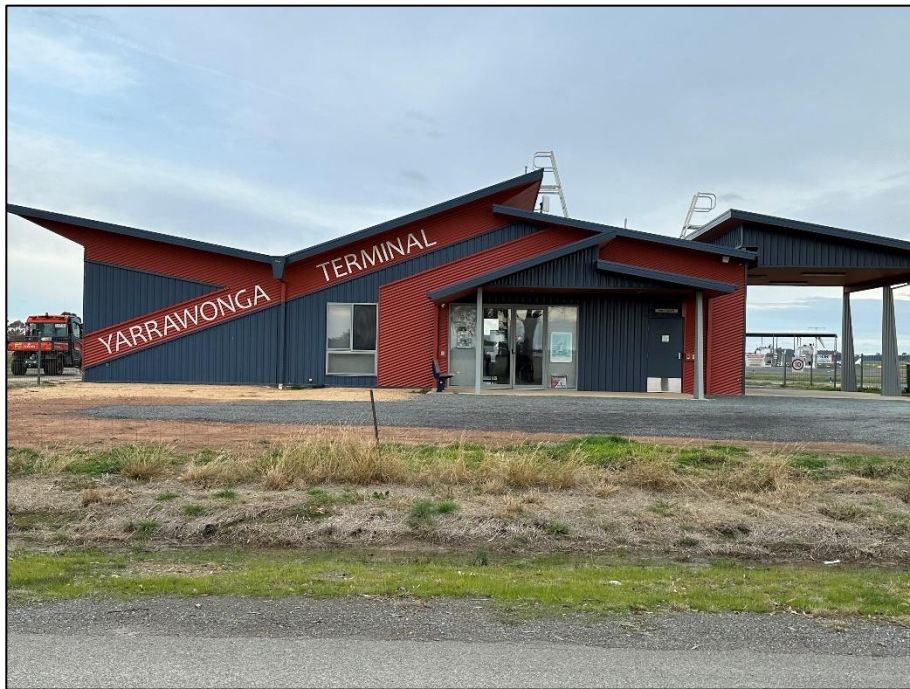
Figure 18 Yarrowonga Terminal building (landside)
