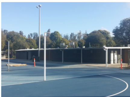
Asset: JC Lowe Oval Netball Change Rooms
