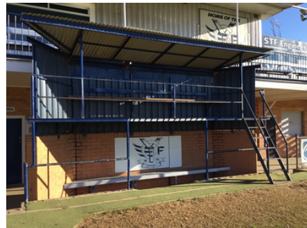
Asset: JC Lowe Oval Interchange Boxes
