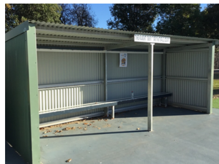
Asset: JC Lowe Oval Netball Shelters
