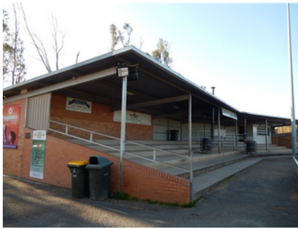
Asset: JC Lowe Oval Grandstand
